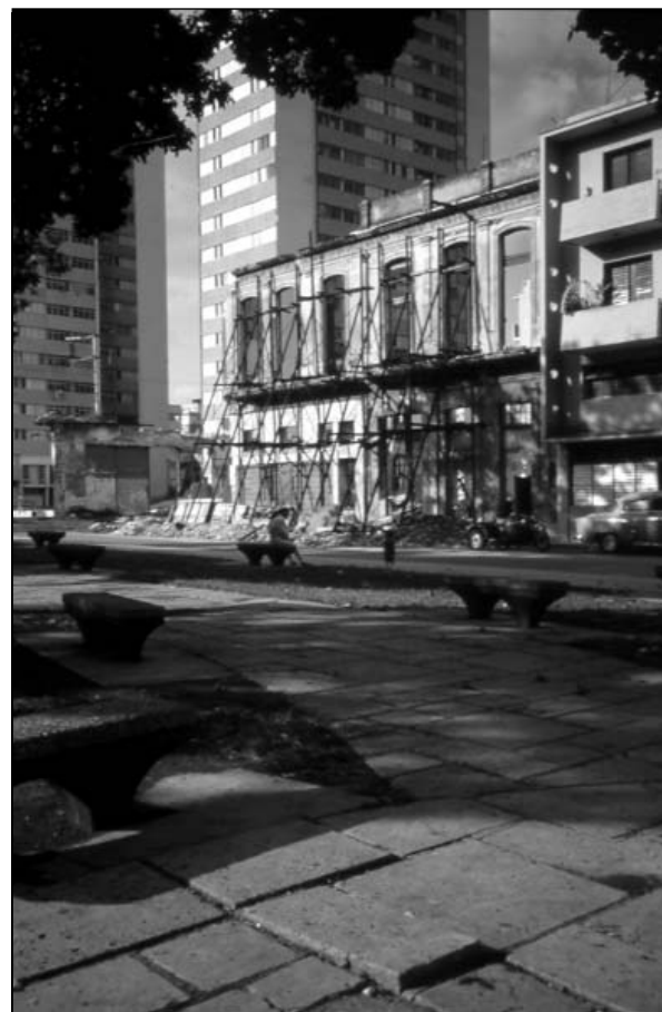
Photo 11: A Neoclassical Façade in Cayo Hueso, Shored Up after the Partial Collapse and then Demolition of the rest of the Building. Behind is a 20-Storey Prefab Apartment Building from the 1970's Urban Renewal Project
