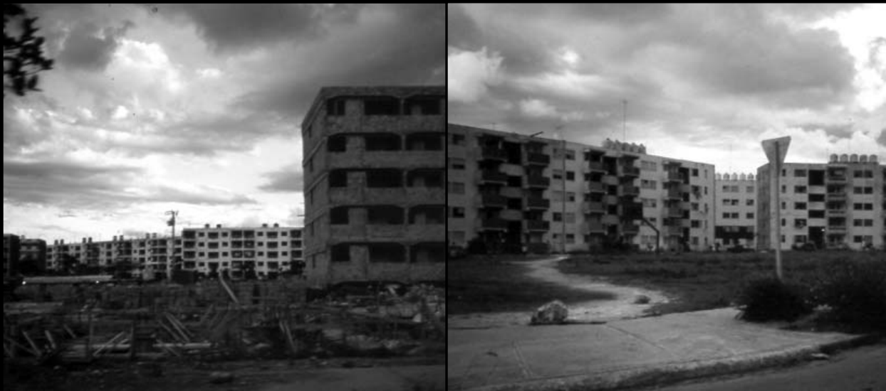
Photo 10. Five-Storey Walk-Ups are Typical of Microbrigade Housing in Alamar
