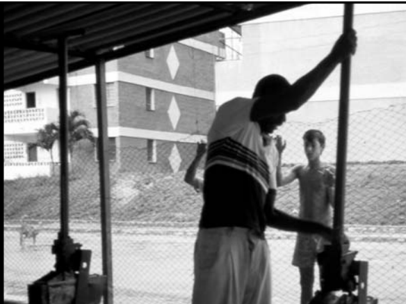
Photo 19. Manual Block-Making Machine Operated in La Güinera, with Five-Storey Standard Semi-Prefabricated Buildings in the Background
