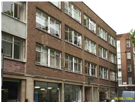
Figure 5. An office building with a high percentage of open windows.
